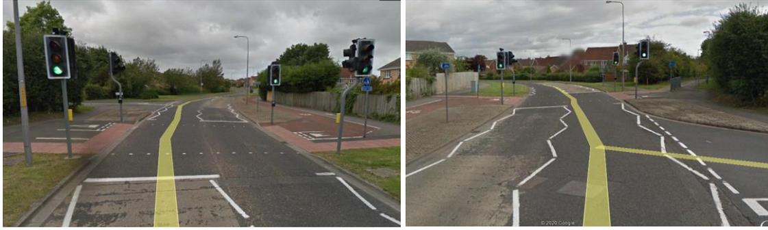
Located on a bend to the east of Challacombe Crescent, the provision of a raised table top at the pedestrian/cycle puffin crossing and the inclusion of an advisory 20mph speed limit would have the effect of slowing traffic on this section of Sober Hall Avenue.
